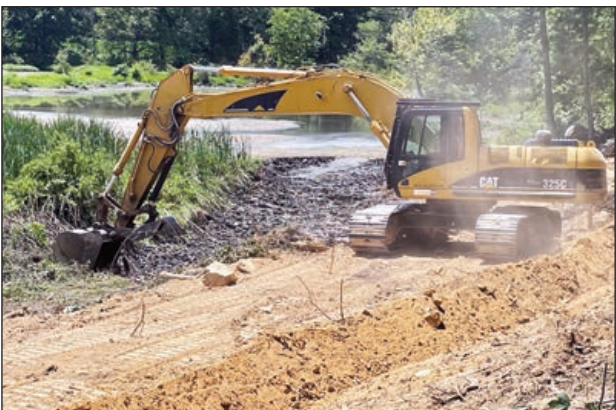
Engineers believe that cutting a new supply ditch from Crooked Creek to Old City Lake will release more water available for treating. Local contractor Shelby Belt with his track hoe was clearing the way for those plans on Monday and Tuesday.
